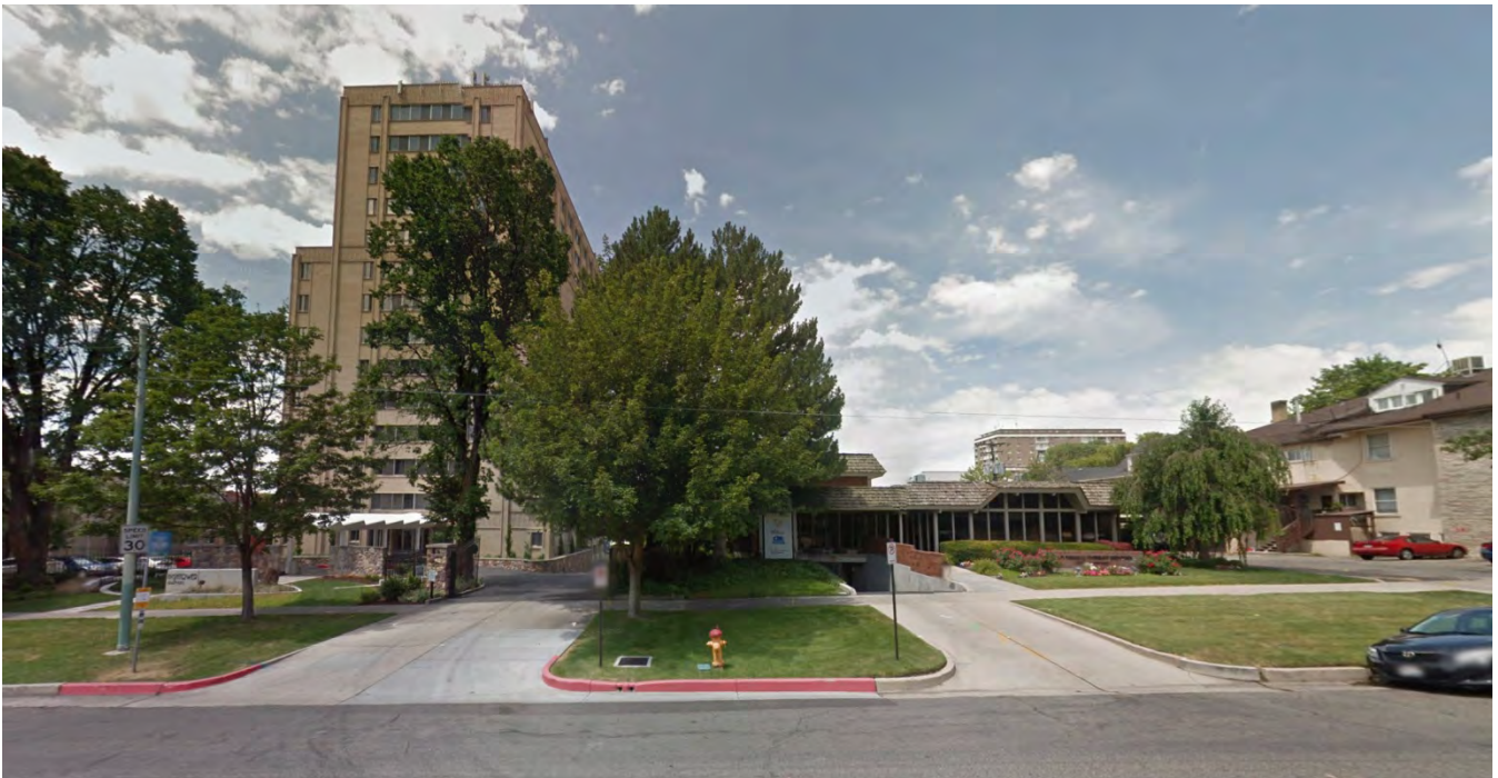
Existing development on the west side of 900 East.
