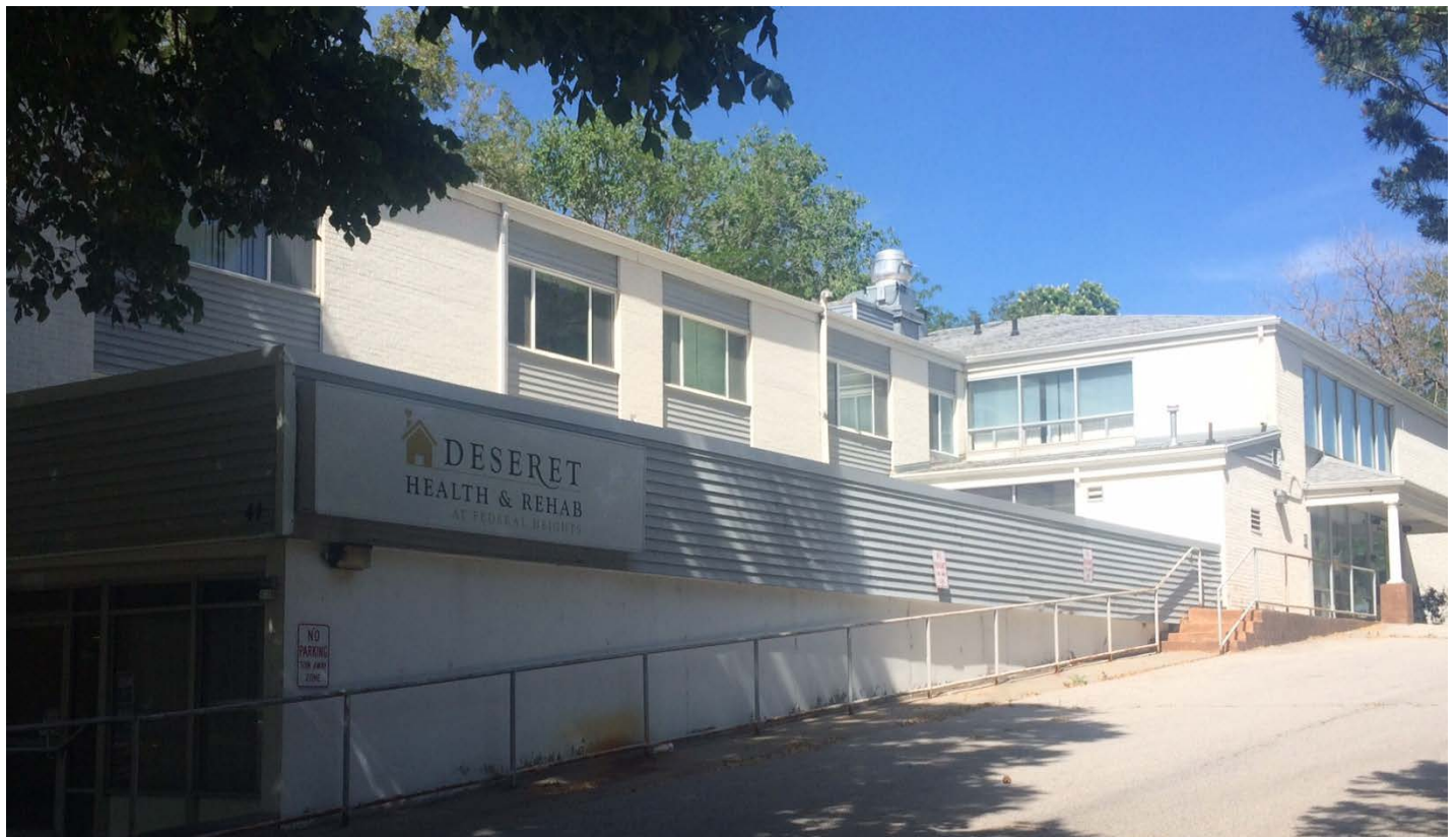
Building located at 57 S 900 East. The slope of the lot increases toward the east (rear of the lot).
